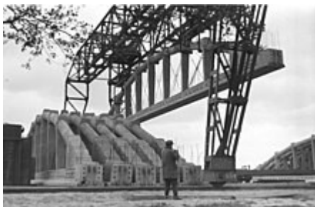
A roof truss of U-bootbunker Valentin is lifted into place (1944)
